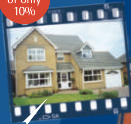
Double Garage converted to an Office retaining Single Garage
